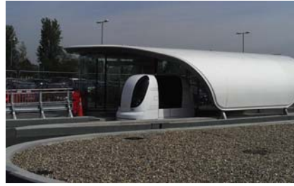
Figure 1. ULTra station and T-Pod at Heathrow
